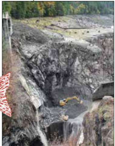
Glines Canyon Dam removal progresses.
