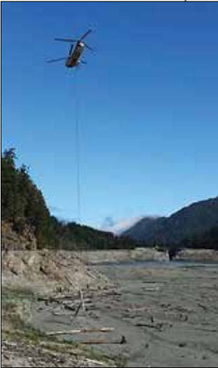
Helicopter transporting woody debris to reservoir bed.
