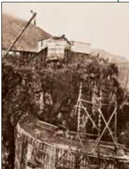
Construction of the Glines Canyon Dam, circa 1925.
