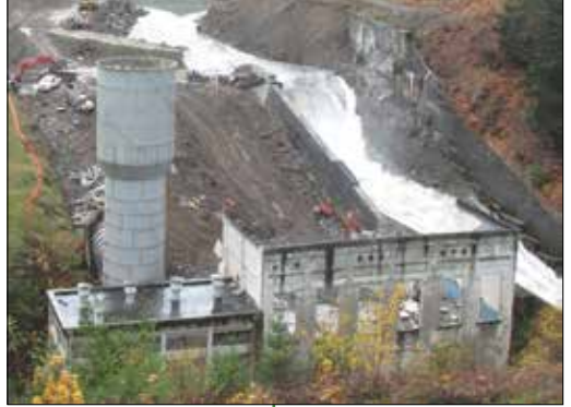
Elwha Powerhouse demolition, 2011.
