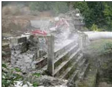
Elwha gravity dam removal.
