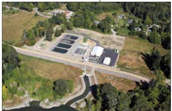
An aerial view of the new Elwha River hatchery, 2011.
