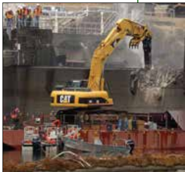
Glines Canyon Dam demolition begins.
