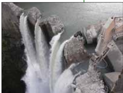
Notching Glines Canyon Dam.
