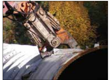
Removal of penstocks.
