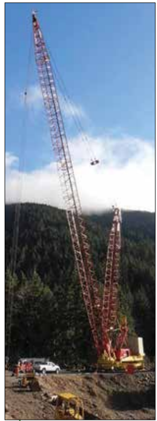
A 200 foot crane at the Glines Canyon Dam site.
